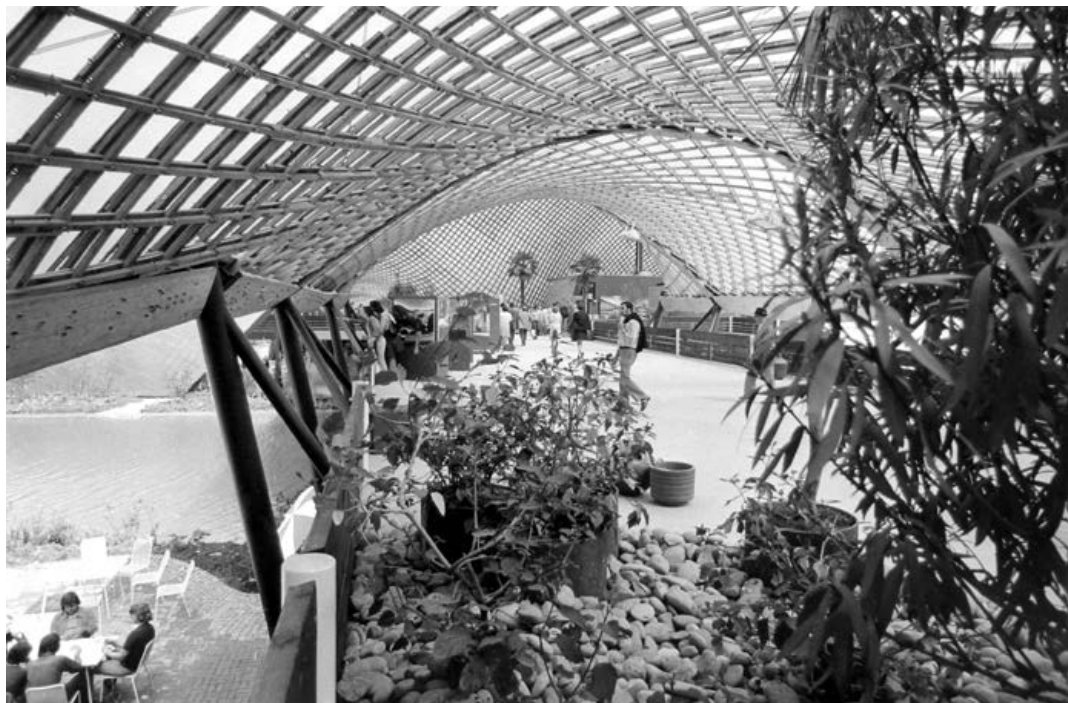
Inside and outside the gridded shell roof covering.
