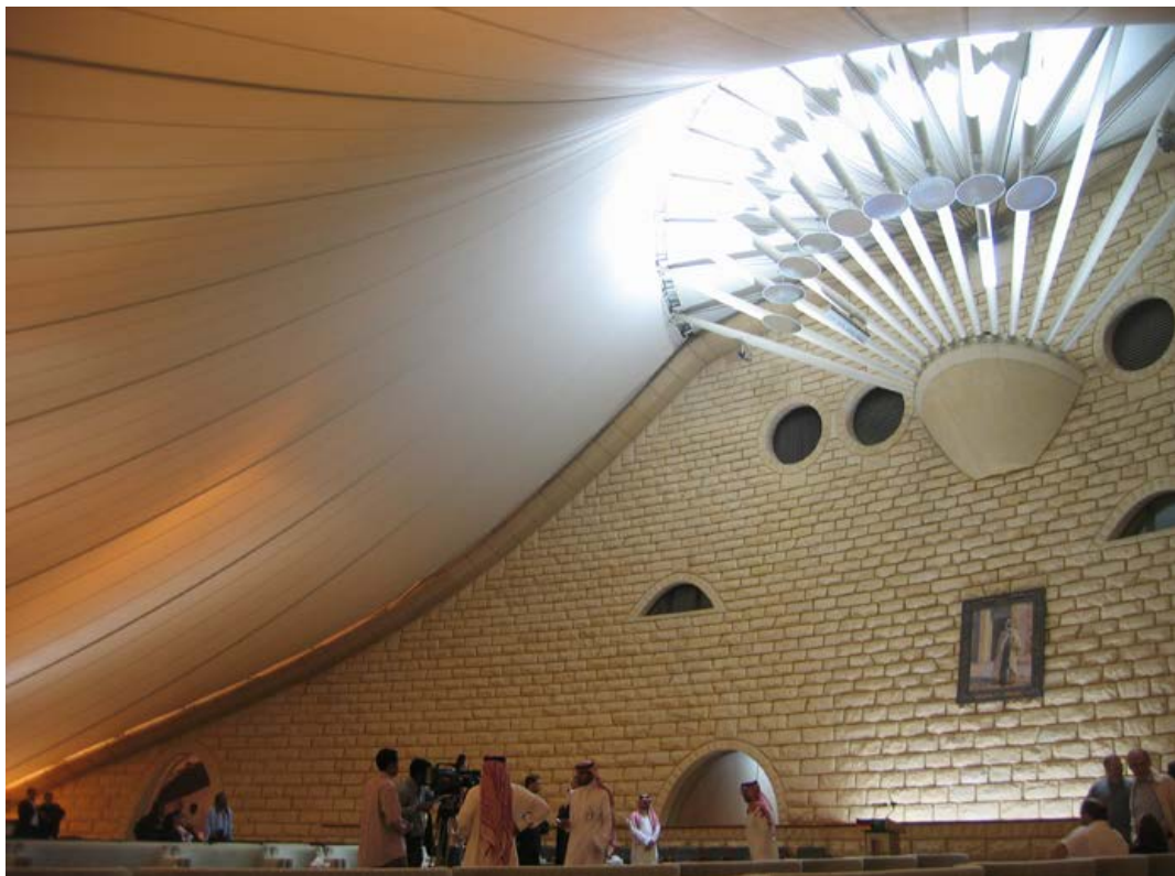
Showing the tent attached to the wall.
