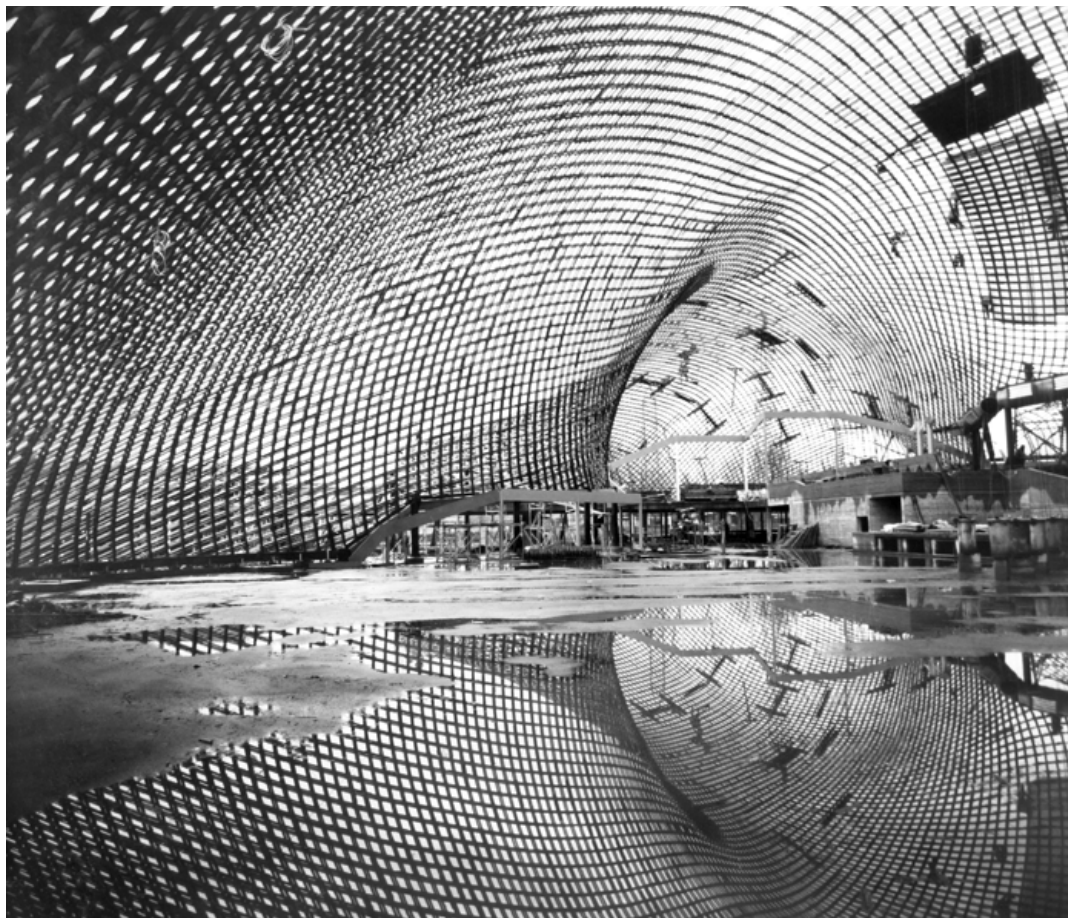
Installing the grid
