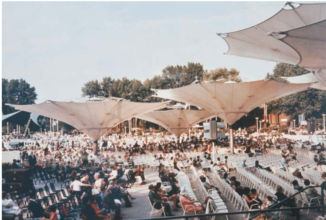
A continuous roof of large overlapping umbrellas.
