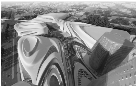
Figure 3. Soehne & Partners, project the Code Unique Hotel in Dubai , 2008 (source: http://www.soehnepartner.com (accessed: 02. 04. 2015)).
