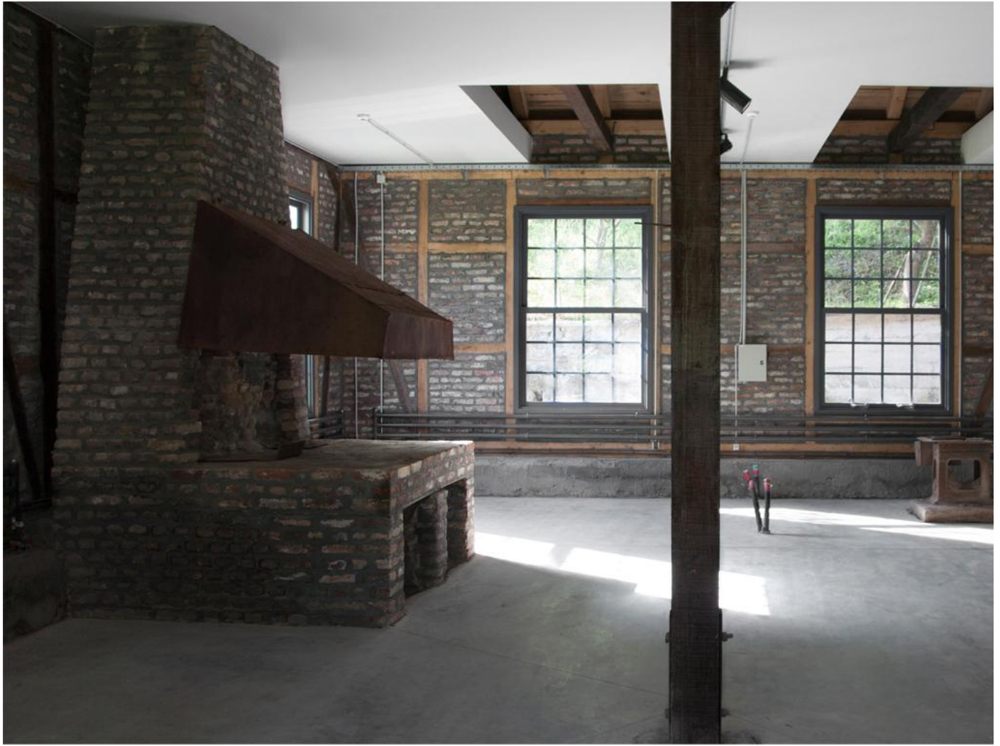
WORKSHOP BUILDING / FORGES ROOM
