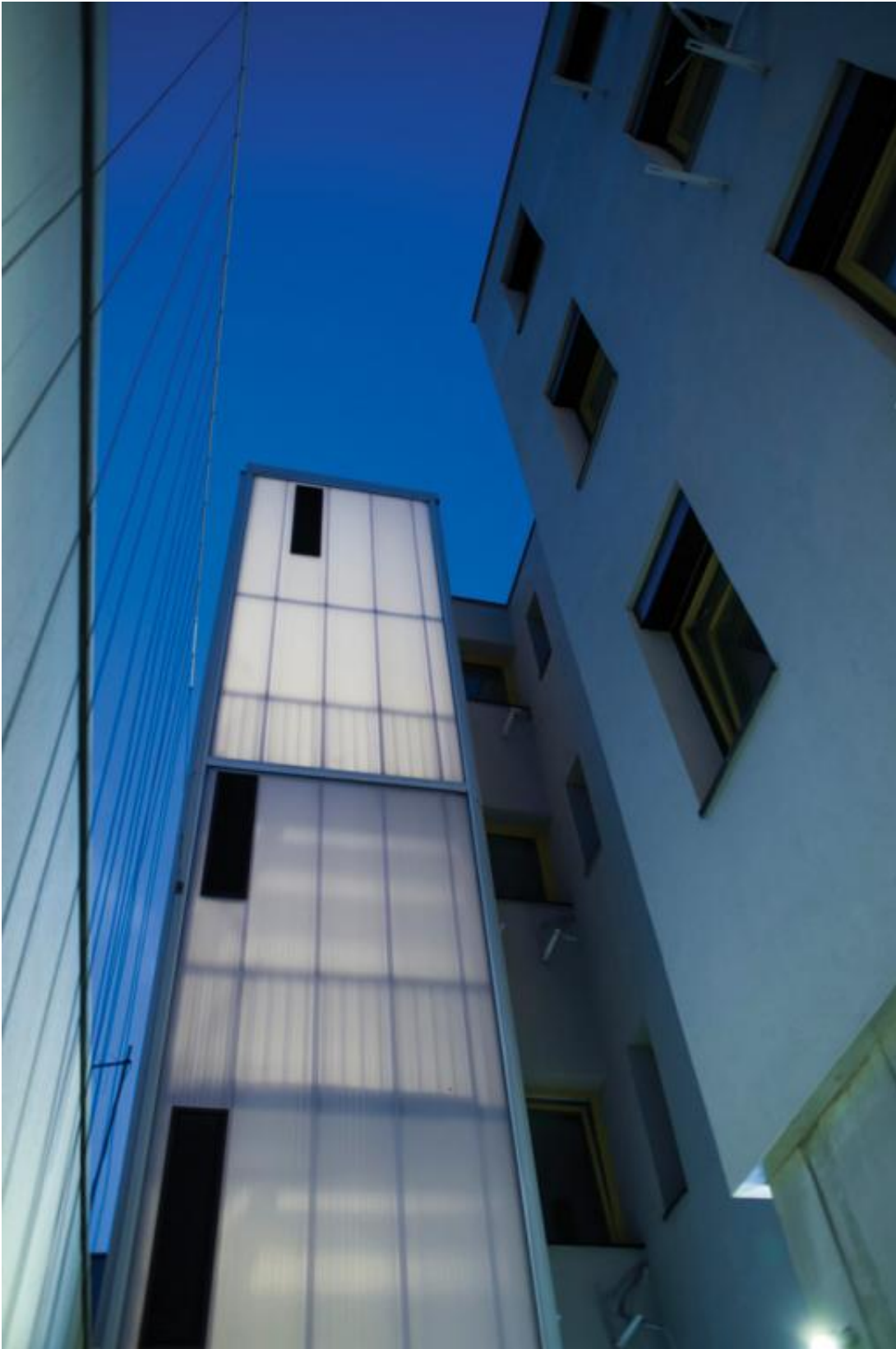
REAR FAÇADE WITH STAIRCASE 1 COVERED WITH LEXAN PANELS WITH BLACK VENTILATION GRIDS
