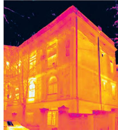
A residential building with massive façade brick walls without thermal insulation. The thermal image shows heat losses evenly distributed through façade walls, particularly intense at horizontal reinforced concrete ring beams. Some windows have been replaced with modern PVC with good thermal performance in contrast to original constructions characterized by noticeable heat loss.
