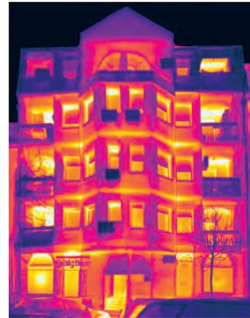
A residential building with a façade realized in a combination of various materials, mostly with inadequate thermal characteristics. The thermal image shows noticeable heat loss at all reinforced concrete ring beams and at connections between terrace slabs and façade walls. Façade fenestration is of relatively poor quality with noticeable heat loss.
