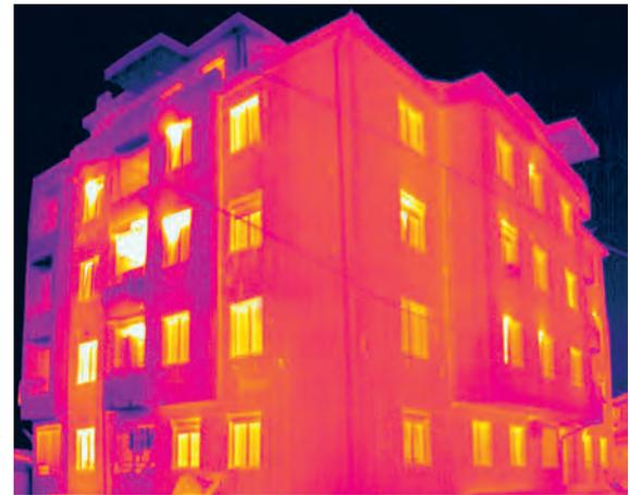
A residential building with massive hollow clay block walls and a contact façade insulation system. The thermal image reveals no noticeable heat loss zones except at façade window constructions and partially at jetty panels. There are spotted heat zones resulting from gaps occurring at installment of thermal insulation panels.
