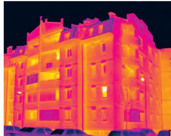
A residential *lamela* building with massive sandwich walls and mortar rendering. The thermal image shows no noticeable heat loss zones except at connections between terrace slabs and façade walls, windows and partially at jetty panels. There is visible façade wall layer pattern as well as colder linear zones resulting from additional insulation of horizontal ring beams and lintels.
