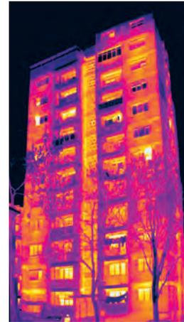
A residential high-rise tower with massive façade walls built of *Durisol* blocks without thermal insulation. The thermal image reveals noticeable heat loss through façade walls, particularly at horizontal and vertical reinforced concrete ring beams. There is intense heat loss through parapet walls so that the positions of heat sources (radiators) are visible. The original façade fenestration has deteriorated, resulting in intense heat loss.
