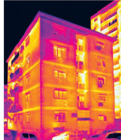
A residential building with massive façade walls built of *Durisol* and concrete blocks without thermal insulation. The thermal image shows noticeable heat loss, particularly at horizontal reinforced concrete ring beams and at the connections between particular blocks; there is also solar heat gain (top floor on the left). Façade fenestration has deteriorated, resulting in intense heat loss.
