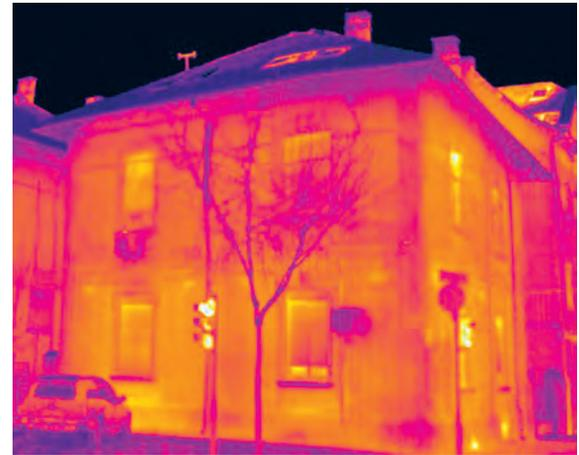
A residential building with massive, homogeneous façade brick walls without thermal insulation. The thermal image shows heat losses evenly distributed through façade walls built without reinforced concrete ring beams. The attic has been subsequently insulated and converted for occupancy. Window constructions show noticeable heat loss.
