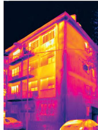
A residential building with massive façade brick walls without thermal insulation. The thermal image reveals intense heat loss through façade walls of the heated section, particularly at horizontal reinforced concrete ring beams, in contrast to the unheated ground floor section. Secondary solar heat gain is noticeable on the upper floors; there are also higher heat losses at façade window constructions.
