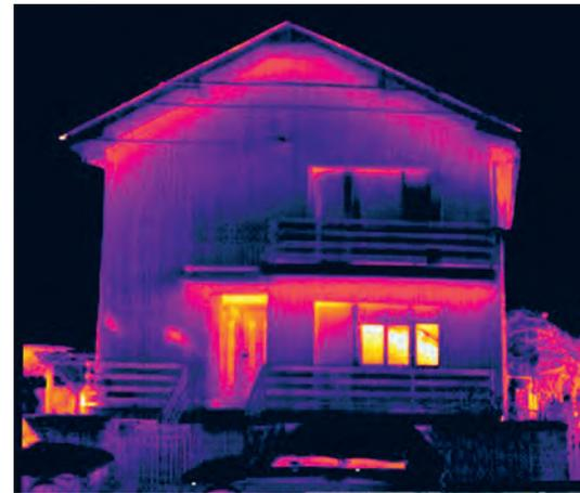
A family house with massive walls and the façade subsequently thermally insulated with a contact façade system using polystyrene blocks. The thermal image reveals heat losses at the points where cantilevered terraces penetrate the thermal envelope and at the eaves zone. The window and entrance door constructions are inadequate, showing noticeable heat loss.
