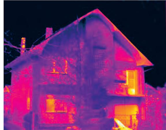
A family house with massive brick walls and subsequent addition of thermal insulation in the rendered façade zone. The window and entrance door constructions are inadequate, showing noticeable heat losses. The house is not entirely heated. The window constructions on the right have higher temperature readings due to solar heat gains.
