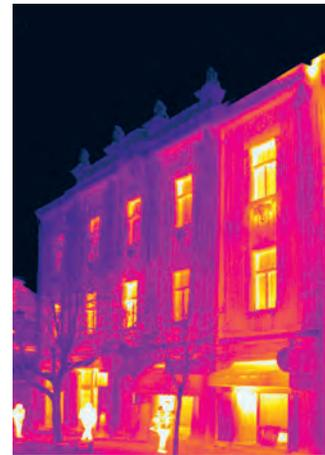
A residential building with massive, homogeneous façade brick walls without thermal insulation. The thermal image shows heat losses evenly distributed through façade walls built without reinforced concrete ring beams. Most windows have been replaced with modern PVC with good thermal performance in contrast to original constructions characterized by noticeable heat loss.
