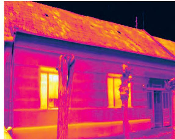
A family house with uninsulated massive brick walls. The house is not entirely heated; the thermal image clearly shows the heated room in the left section of the front façade. There is noticeable solar heat gain on the roof surface. The window construction is inadequate, showing extensive heat loss especially at roller shutter boxes.
