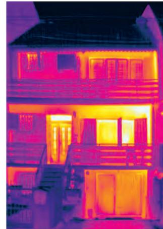
A family house in a row with uninsulated massive façade walls made of brick. The entire house is heated; the thermal image reveals a clear contrast with the unheated attic area. The most noticeable heat losses occur in the zones of reinforced concrete ring beams and lintels. The window and entrance door constructions are inadequate, showing significant heat loss.
