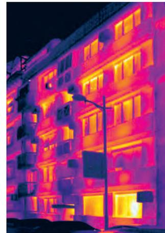
A residential building with a façade realized in a combination of various materials, mostly with inadequate thermal characteristics. The thermal image shows noticeable heat loss at reinforced concrete ring beams and window constructions, especially at roller shutter boxes. There is intense heat loss through uninsulated façade brick parapets with visible positions of heat sources – radiators.
