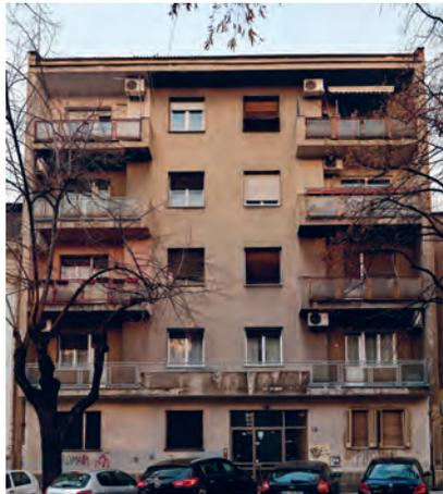
A residential lamella building with massive façade brick walls without thermal insulation. The thermal image shows different intensities of heat loss through façade walls at reinforced concrete ring beams and wall infill. There is also a noticeable contrast between the unheated attic and ground floor unit, and the heated section of the building. Façade fenestration is characterized by intense heat loss.
