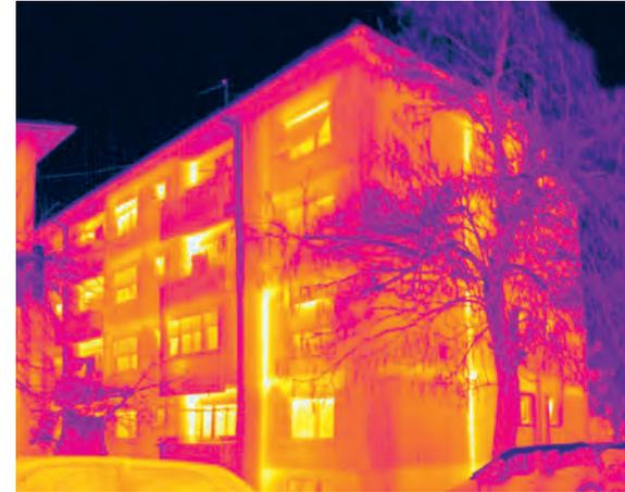
A residential building with massive façade brick walls without thermal insulation. The thermal image reveals noticeable heat loss through façade walls, particularly at horizontal reinforced concrete ring beams, lintels and cantilevered terraces. The original façade fenestration has deteriorated and reveals intense heat losses at frame connections and roller shutter boxes.
