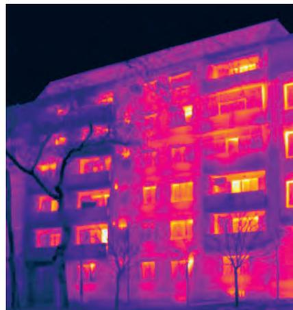
A residential building with massive façade brick walls without thermal insulation. The thermal image reveals noticeable heat loss through façade walls, particularly at horizontal reinforced concrete ring beams, lintels and cantilevered terraces. The original façade fenestration reveals intense heat losses at frame connections and roller shutter boxes.
