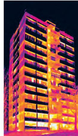
A residential high-rise tower with uninsulated full façade concrete or breezeblock walls and alternating ribbons of light parapet walls and windows. The thermal image shows noticeable heat losses through lateral massive walls, especially at ring beams and connections between parapet walls and windows. Due to high reflectivity, the metal parapet cladding shows unrealistically low temperature readings.
