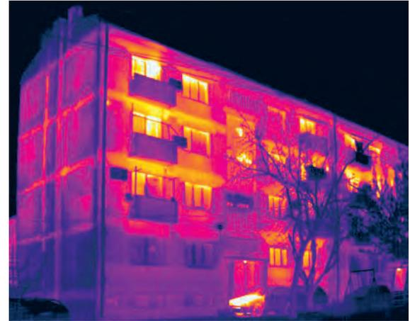
A residential *lamela* building with massive façade brick walls without thermal insulation. The thermal image shows different intensities of heat loss through façade walls at reinforced concrete ring beams and wall infill. There is also a noticeable contrast between the unheated attic and ground floor unit, and the heated section of the building. Façade fenestration is characterized by intense heat loss.
