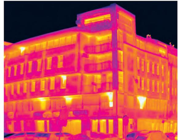
A residential building with a complex façade realized in a variety of materials. The thermal image shows noticeable heat loss at horizontal and vertical reinforced concrete ring beams, connections between terrace slabs and façade walls, and jetty panel overhangs. In places, there are intense hot zones resulting from open windows.
