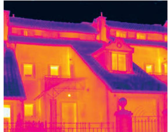
A family house in a row with massive hollow clay block façade walls, brick cladding, and thermal insulation. The entire house is heated; the thermal image shows uniformity and no distinctive linear losses. Thermal performance of the walls and window and door constructions complied with the thermal regulations of its time.
