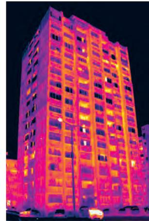
A residential high-rise tower with façade walls built of prefabricated concrete panels. The thermal image shows heat loss at connections between panels and within their structure: connections between load bearing and final layers, especially parapet elements. Intense linear heat loss is characteristic at connections between terrace slabs and façade walls. Façade fenestration is of poor quality and shows noticeable heat loss.
