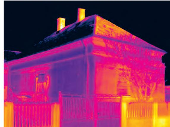
A family house with massive façade brick walls without thermal insulation. The house is not entirely heated; the thermal image clearly distinguishes the heated room in the middle section of the façade on the left. Homogeneous walls are without concrete ring beams and show heat losses evenly distributed over the surface. On the south side, the roof, the façade on the right and especially the concrete fence show solar heat gain.
