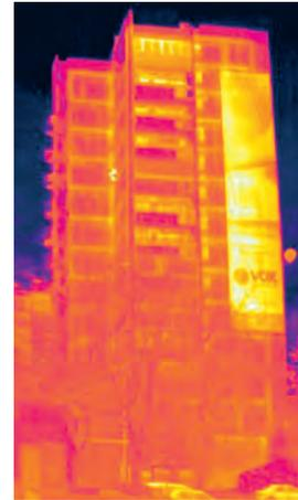
A residential high-rise tower with façade walls built of prefabricated concrete panels. The thermal image shows heat loss at connections between various panels and especially at connections between load bearing and final layers within the same panel. Linear heat loss is characteristic at connections between terrace slabs and façade walls. Façade fenestration is of poor quality and shows noticeable heat loss.
